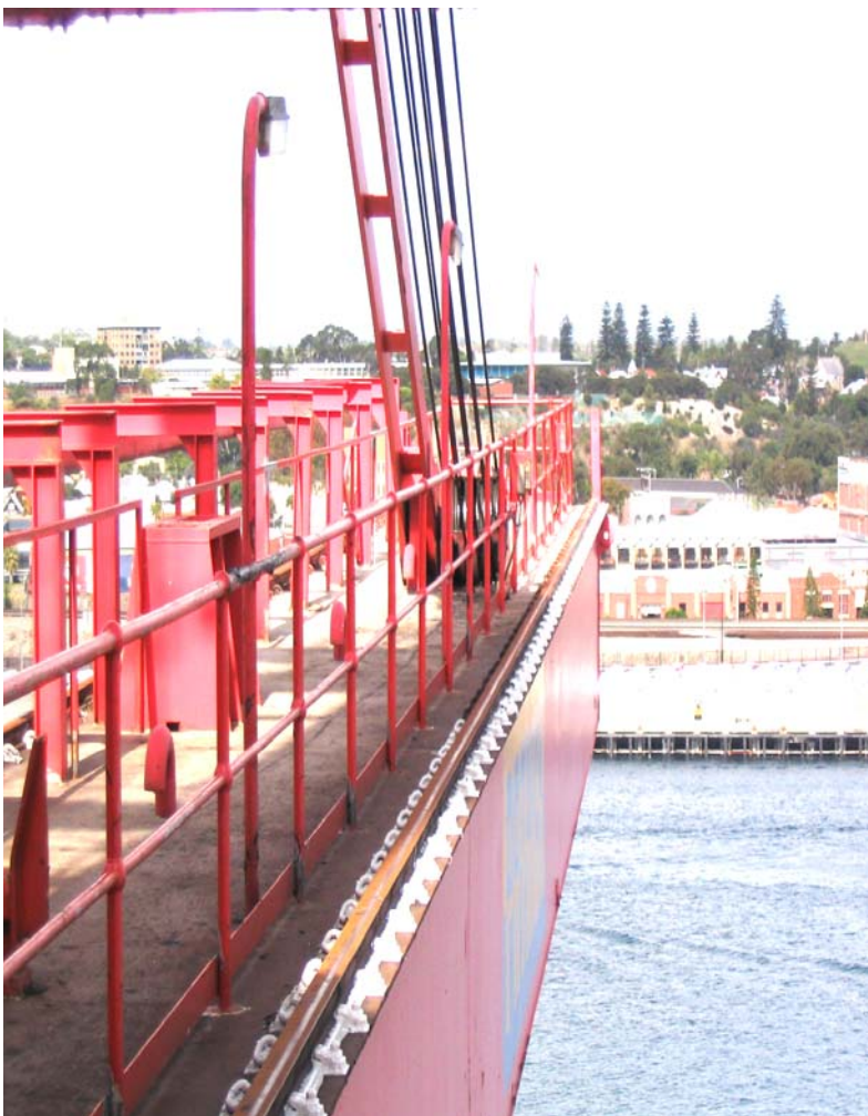
Top: A single cleat and pigtail prior to coating Above: Cleat and pigtail after being coated with Enviropeel Right: A length of track on the jib showing coated cleats linked with Enviropeel to improve security Below Right: Views of Enviropeel coated cleats
