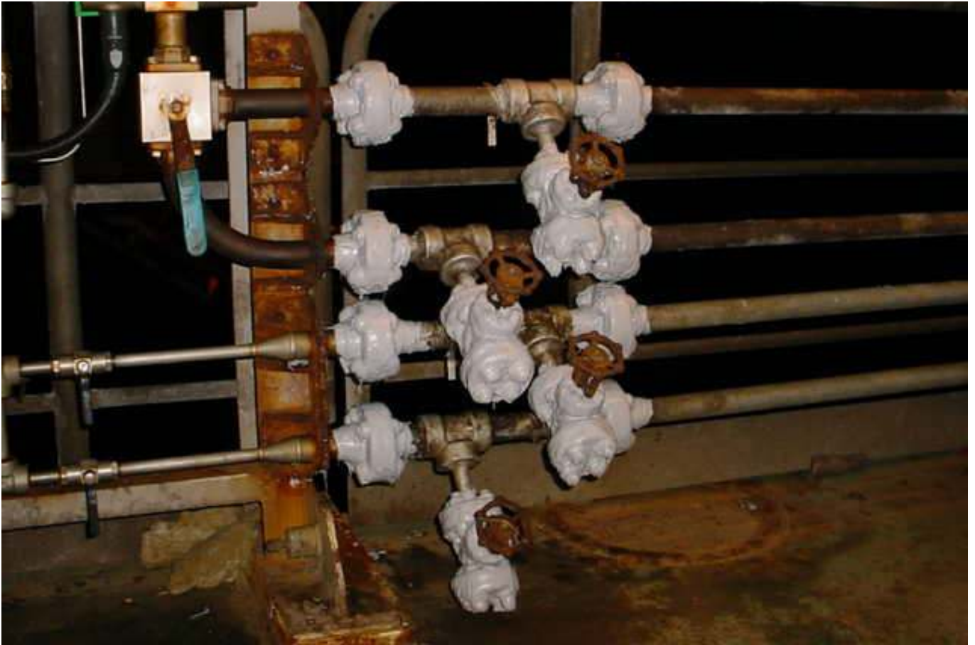
A variety of flanges that have been coated with E170 Grey.
