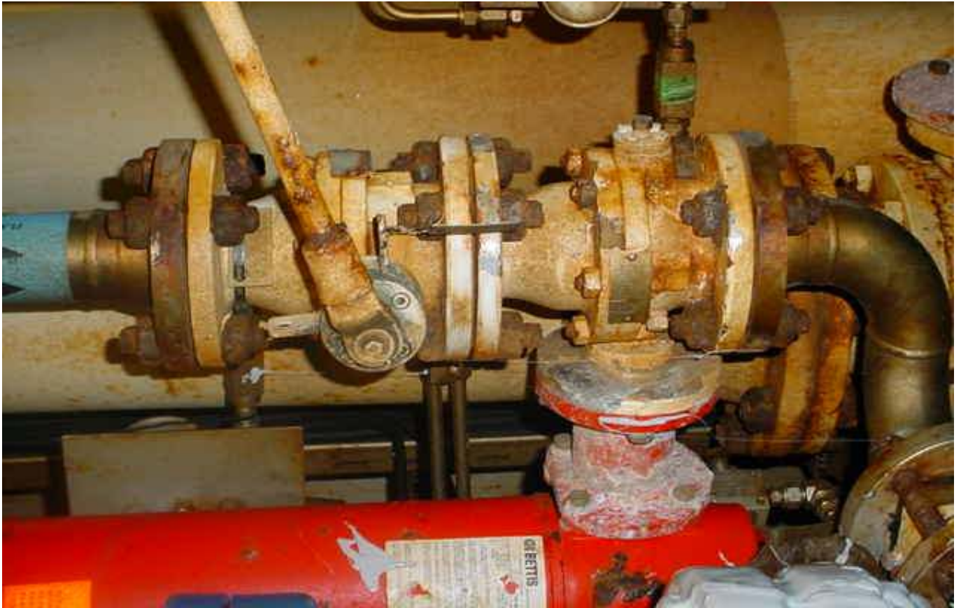
Above: valves and flanges prior to preparation. Below: valves and flanges prepared by hand and ready for application.
