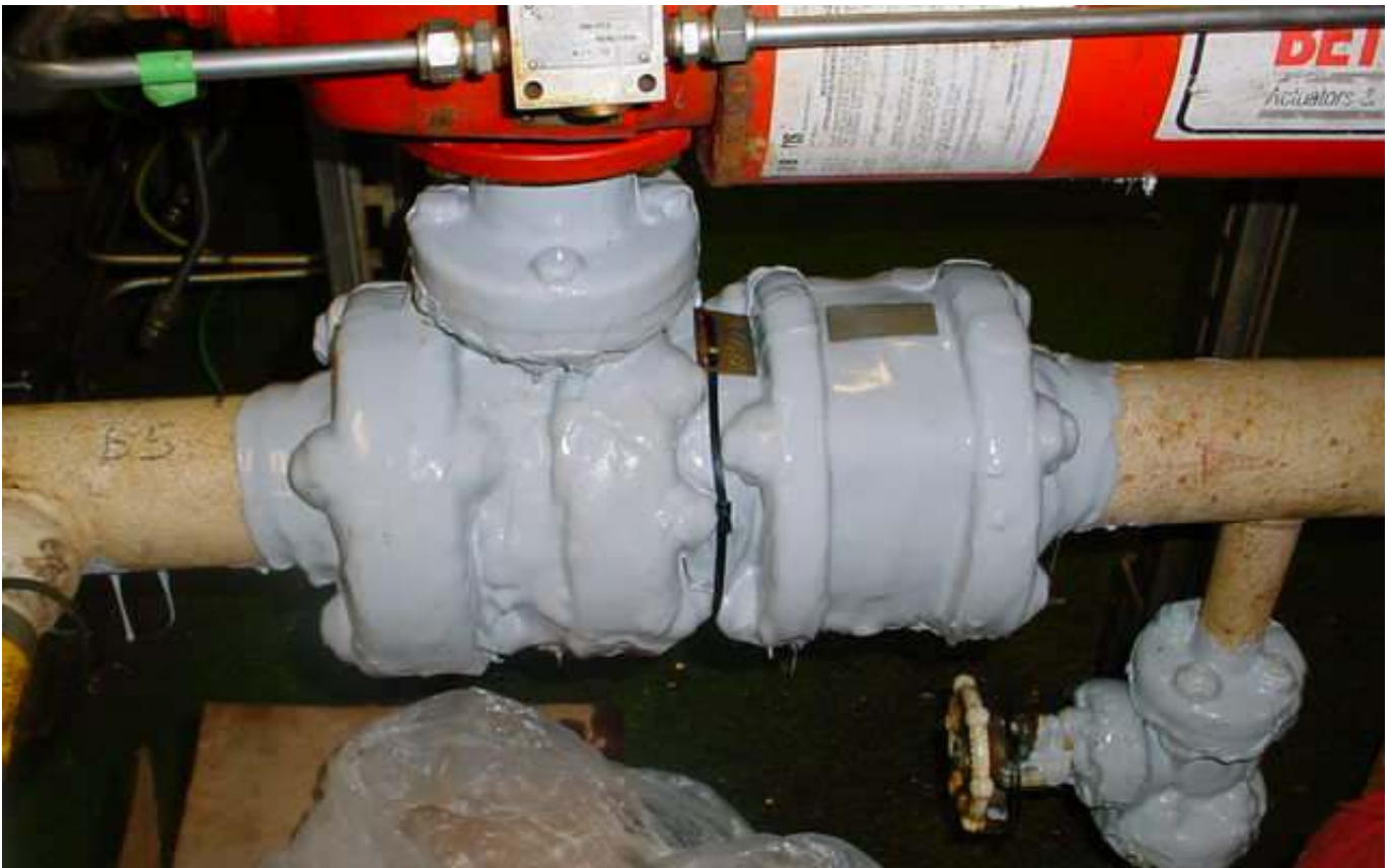
More flanges and valves that have been coated with E170 Grey.
