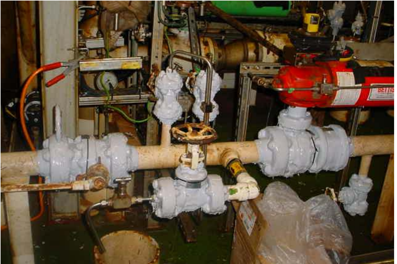
More flanges and valves that have been coated with E170 Grey.
